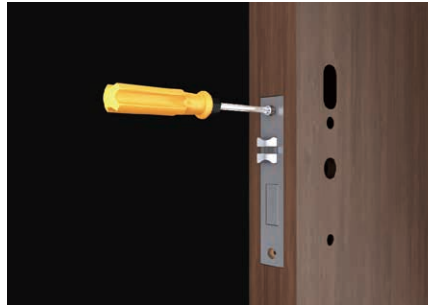
2. Install the inner panel into the door frame Tighten the fixing screw of lock body.
